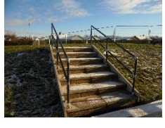
Nosings required and highlight handrails
